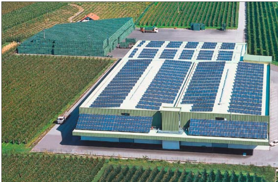
Solar power a la Italiana: a Leitner Solar 272 kW p PV system on the fruit cooperative building of Bozen
